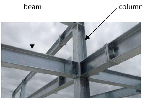
The **columns** are the parts that run **vertically** and the **beams** are the parts of the structure that run **horizontally**. A beam is used to span a gap and is supported by columns on either end.
